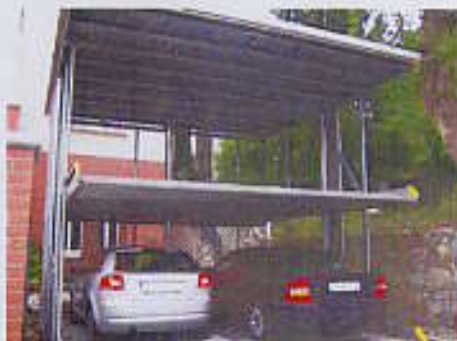
2 cars parked on lower level . 2 cars can be parked on roof plus 2 on upper deck
