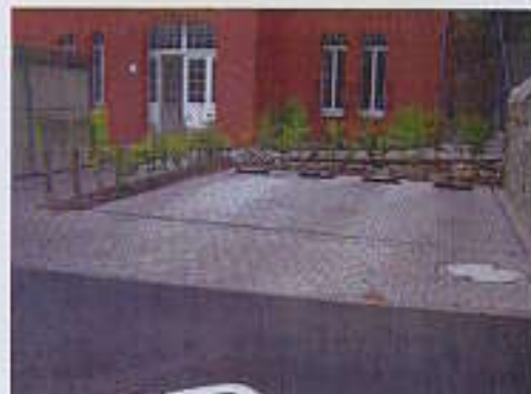
Stacksafe with no parked on roof. 2 or 4 cars can be parked on decks below ground level
