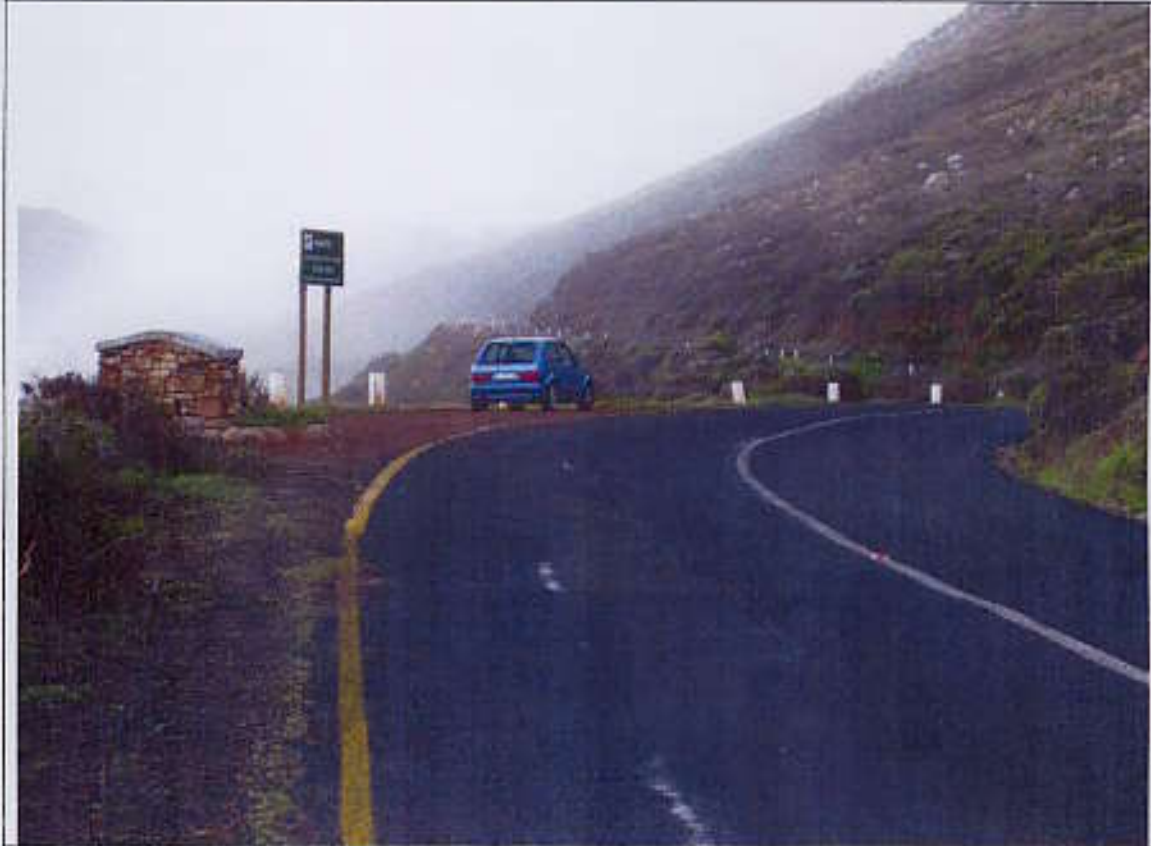
Figure 2.2: North-west Along Main Road From Erf974/1 Towards Parking Area
